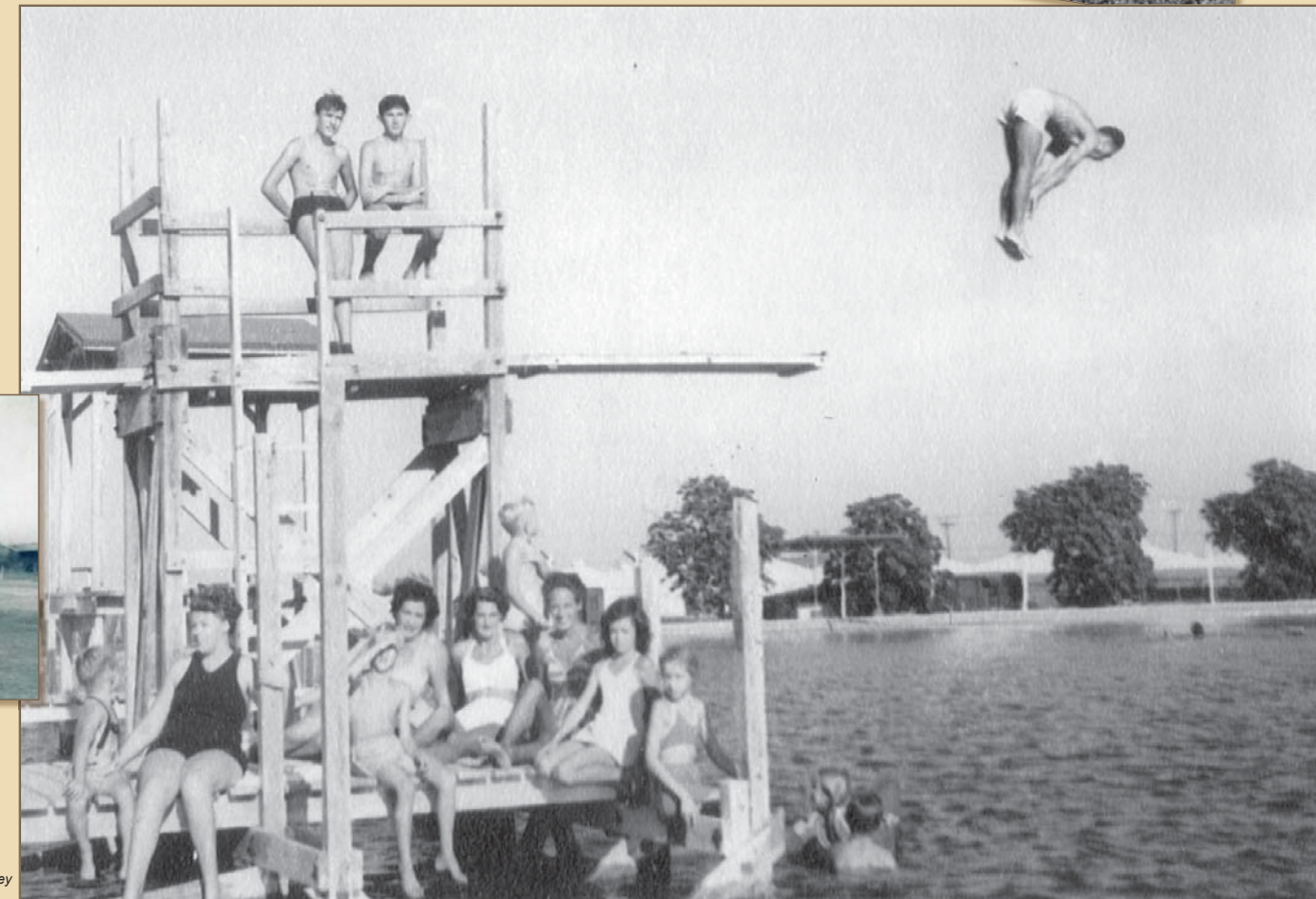
German American internees building the Camp Swimming Pool/Irrigation Reservoir, Institute of Texan Cultures, UTSA, #098-0995, courtesy of Betty Fly.
